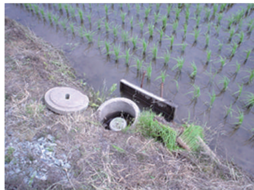
Fig. 1. Automated irrigation gate installed on pressurized irrigation pipe and application example photo(Source: Toshiaki Iida, The University of Tokyo, PAWEES 2016 Conference, Daejeon, Republic of Korea)
