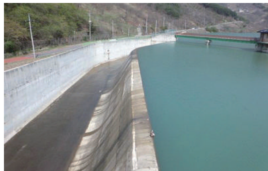
(b) Panorama of chute spillway
